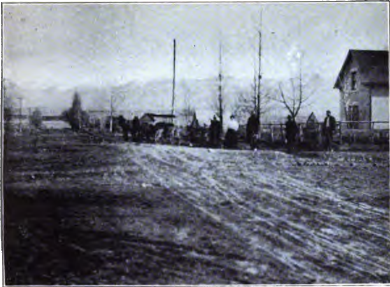
FIG. 13. ROAD IN CHESTER WHERE CITIZENS CONTRIBUTED ALL THE LABOR FOR CONSTRUCTING AND MAINTAINING MANY MILES OF HIGHWAY
